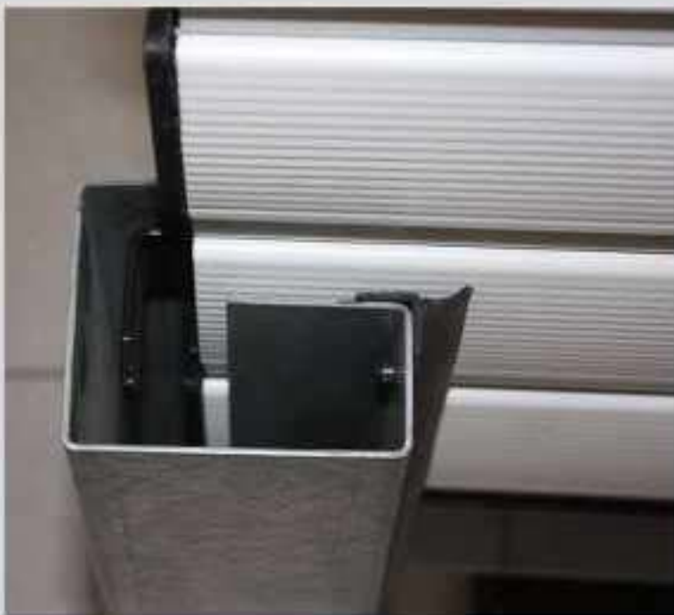
G-shaped rail with tear-proof bracket
