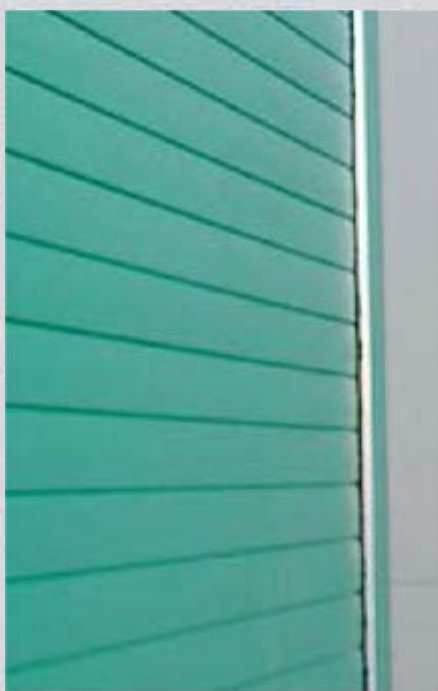
Detail of a guide and relative gasket
