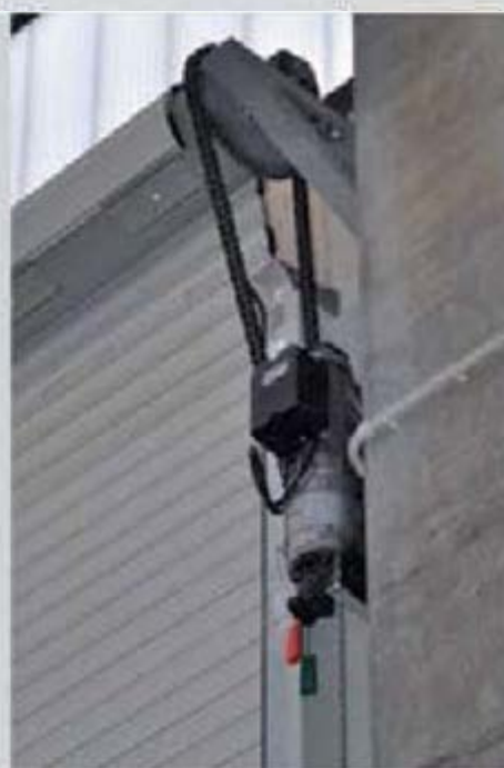
Chain drive side motor
